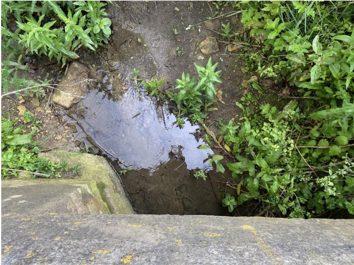
Plate 1 Culvert located at Crossing 1
